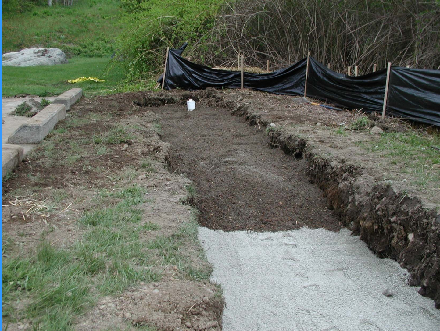
Placement of Bioretention Soil Mix
